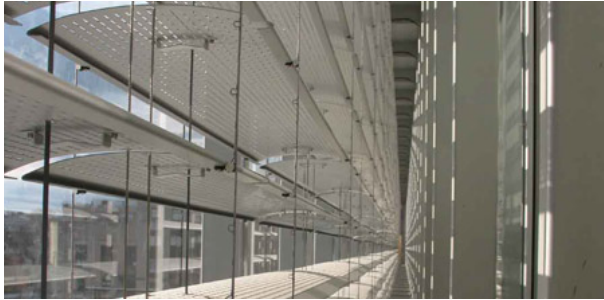
Low-e high performance glass, combined with solar fins to bring in light and prevent solar gains.
