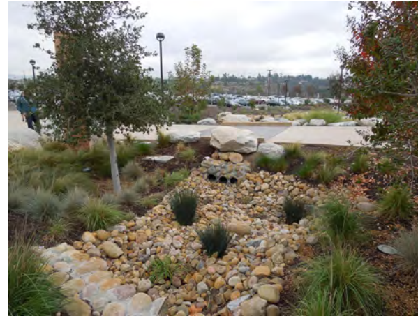
Storm Water Rock Drainage 'Swale' at Grossmont College
